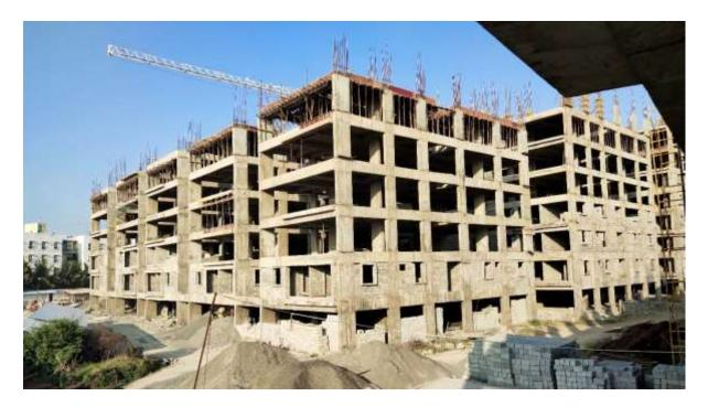
Block D1: : Third Floor level slab First half concrete 100% completed. Shuttering & barbending works in second half of third floor level slab 10% completed and balance work on progress.
