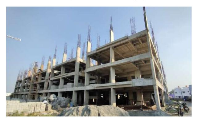
Block A2: Second Floor Level slab concrete casting 100% completed. Barbending work for Column at Second floor on progress
