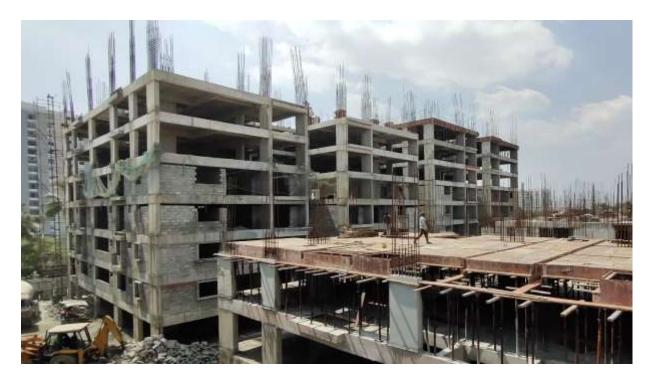
Block D3: Shuttering and barbending work on progress for First half of Sixth floor level slab 85% completed and balance work on progress.
