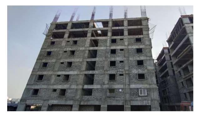
Block C2: Column casting upto Eight floor level 80% completed. Shuttering and barbending works in Eight floor level slab 80% completed and balance works on progress.
